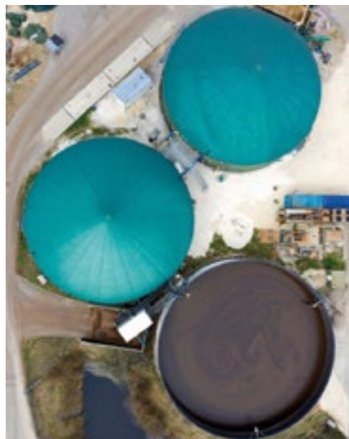
Biogasanlage Foto: iStockphoto.com/Bim
